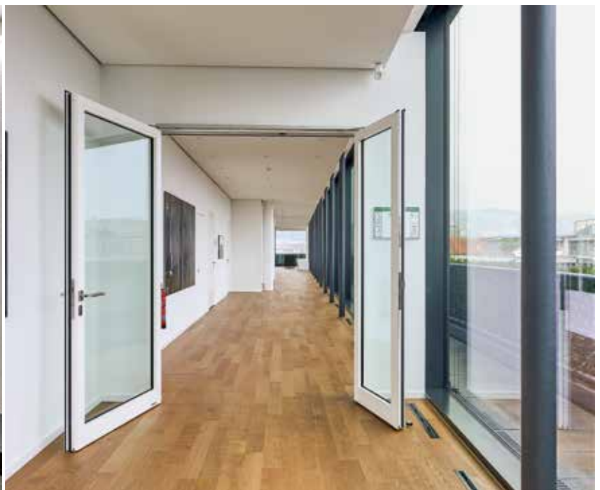
To ensure a maximum clear passage width, the fixed leaf can also be opened up.
