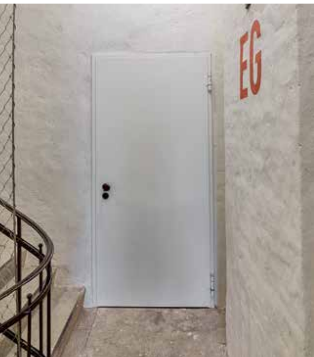
Fire protection in the stairwell with steel doors.
