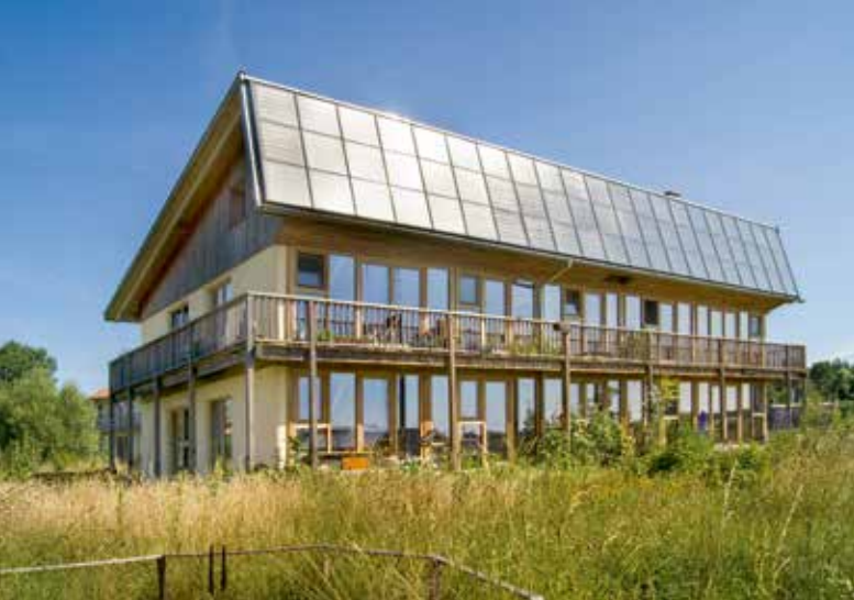
An alternative to conventional construction methods? The building shell of most of the houses in the Sieben Linden ecovillage consists of timber frames, straw and clay plaster.
