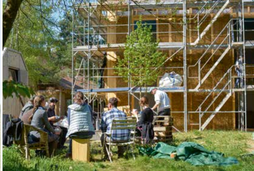
An alternative to conventional construction methods? The building shell of most of the houses in the Sieben Linden ecovillage consists of timber frames, straw and clay plaster.
