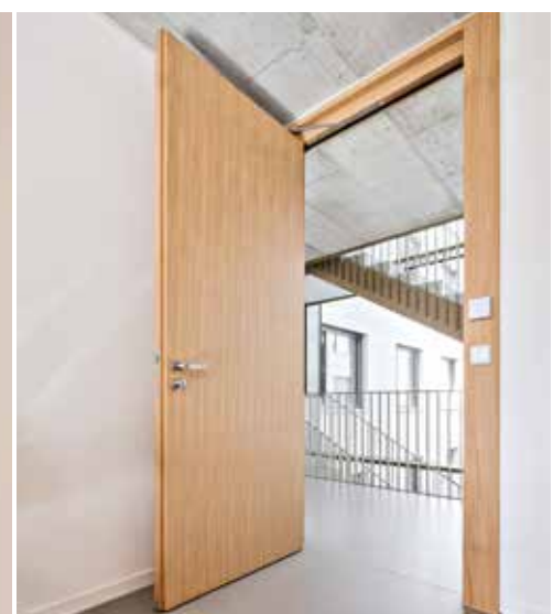
Integrated switch boxes within the door frame.
