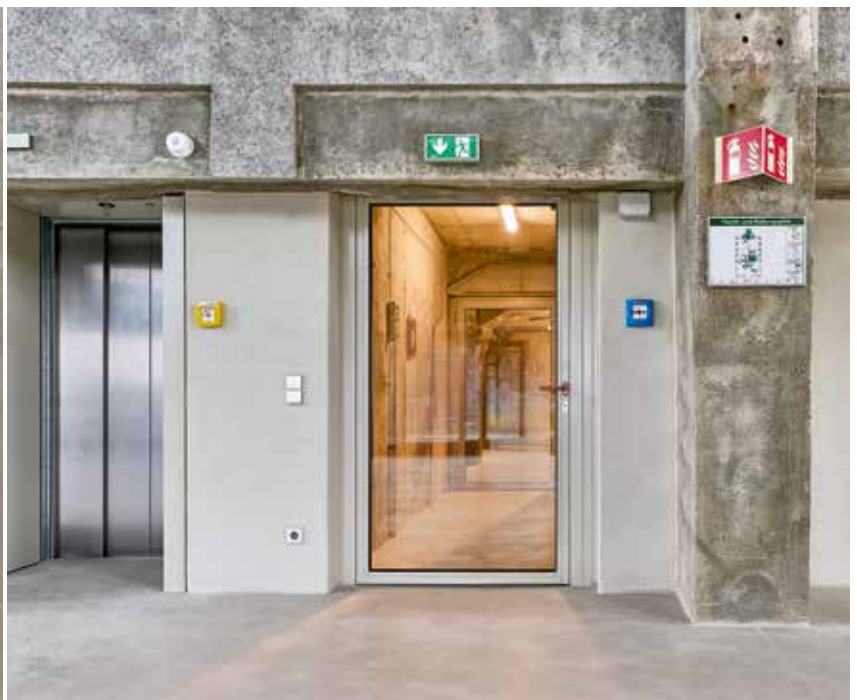
Fully glazed T30 aluminium tubular frame construction project doors are fitted in the "Kornversuchsspeicher" warehouse.
