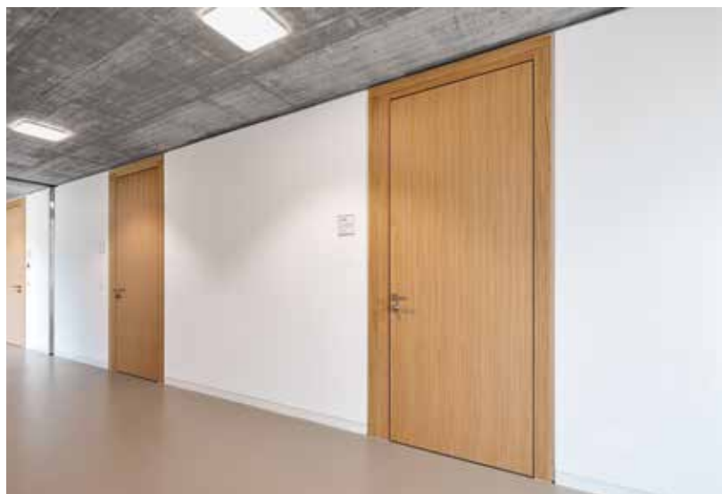
The doors in the Zell town hall are designed to be ceiling-high. A flexible ceiling connection prevents compression when the ceiling bends.
