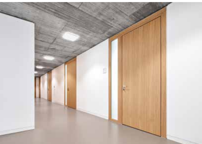
The doors in the Zell town hall are designed to be ceiling-high. A flexible ceiling connection prevents compression when the ceiling bends.
