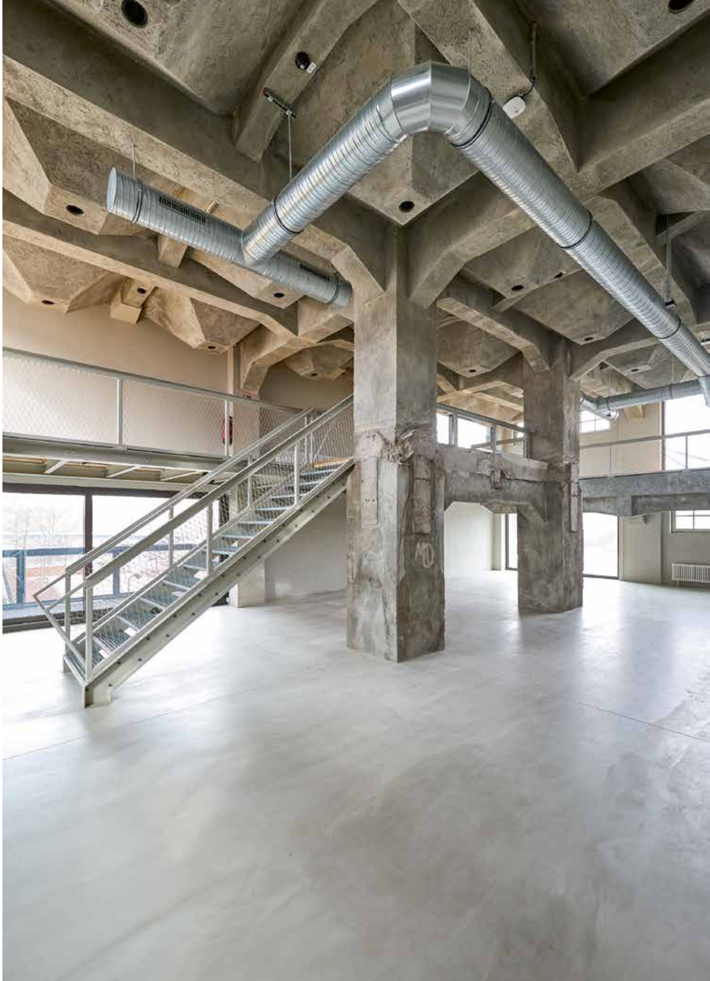
The chutes and their massive reinforced concrete structure are the defining design element in the interior.
