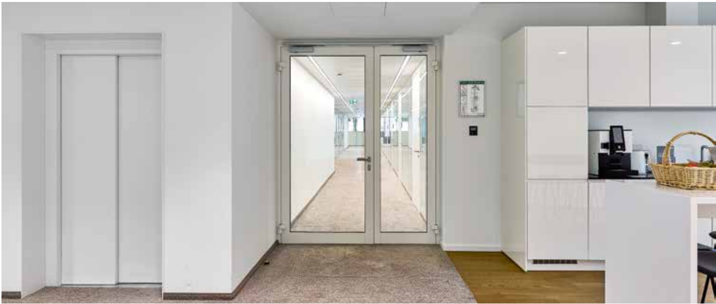
The fully glazed T30 aluminium tubular frame construction project doors allow natural light to enter the interior and ensure good visibility.
