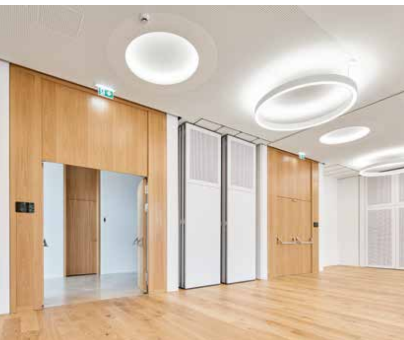
The double-leaf doors in the conference room are fitted with anti-panic levers.
