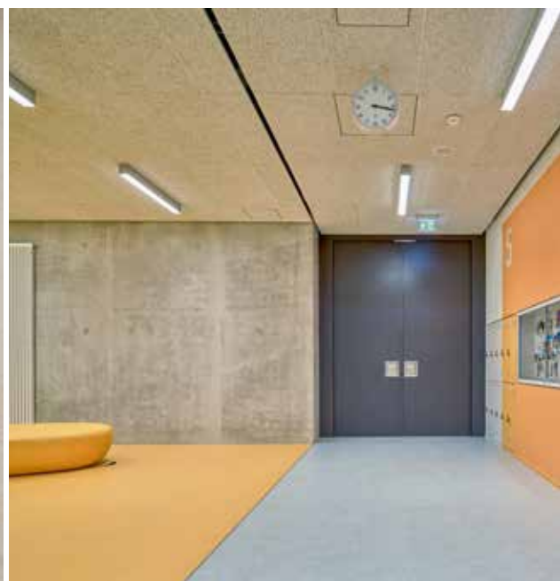
Recessed doors separate the different fire zones and normally only close in the event of a fire. Recessed handles prevent obstruction in everyday life.
