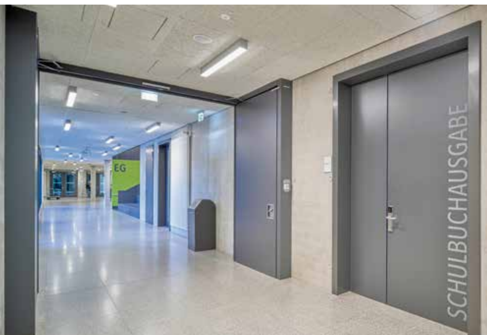
Recessed doors separate the different fire zones and normally only close in the event of a fire. Recessed handles prevent obstruction in everyday life.
