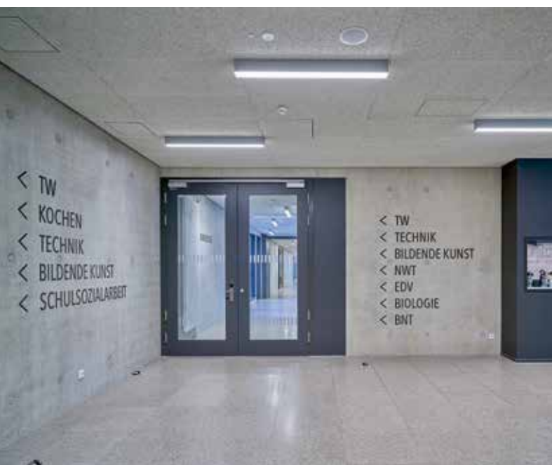
The double-leaf fire-rated doors in the corridor and stairwell also have glazing cut-outs.
