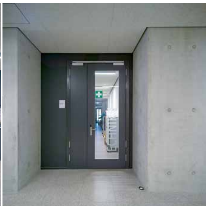
Recessed doors separate the different fire zones and normally only close in the event of a fire. Recessed handles prevent obstruction in everyday life.
